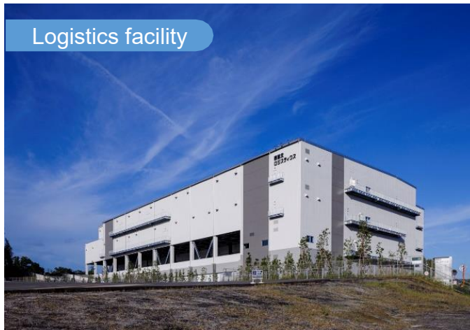
Nishinomiya-kita Logistics Hyogo Prefecture
