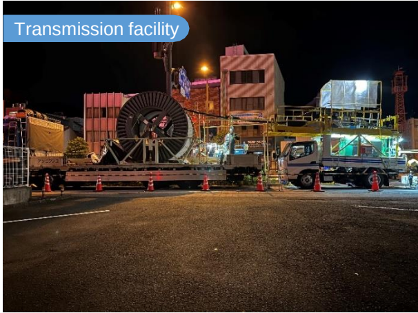
Kuramoto Aiba line and other cables (underground transmission line replacement) Tokushima Prefecture
