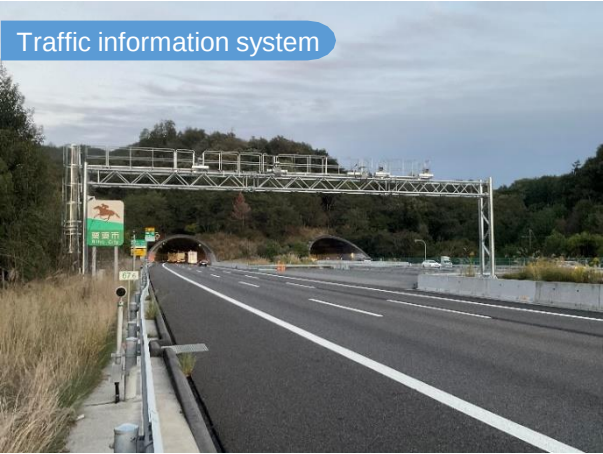
Wireless free flow system in the eastern area of the Kansai Region Shiga, Kyoto, and Osaka Prefectures
